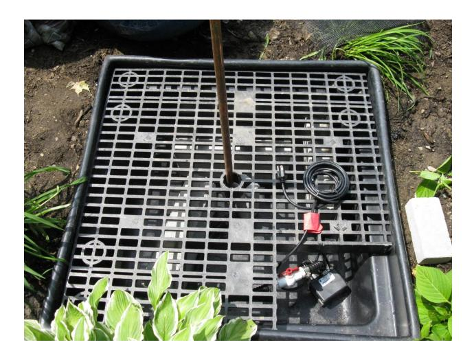
I lowered the basin ppot over the standoff pipe and used my level to hold it plumb. Marine epoxy was then used to secure the pipe to the pot and make it able to hold water.
