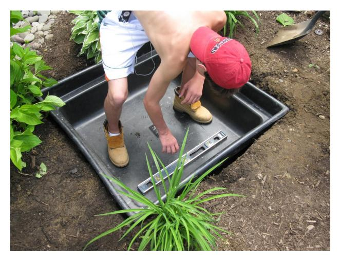
Once the hole was excavated and leveled we installed the reservoir, checked again for level and back filled and tamped. [note: level not shown properly, hold level on edge]
