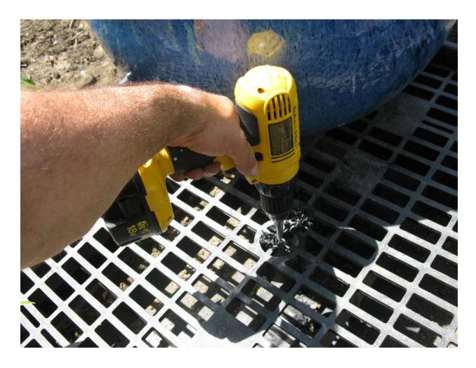
Next step was to drill a hole through the reservoir basin grate for the copper standpipe to reach the reservoir and pump. I used a 1" Forstner bit for this but a spade bit would work too.
