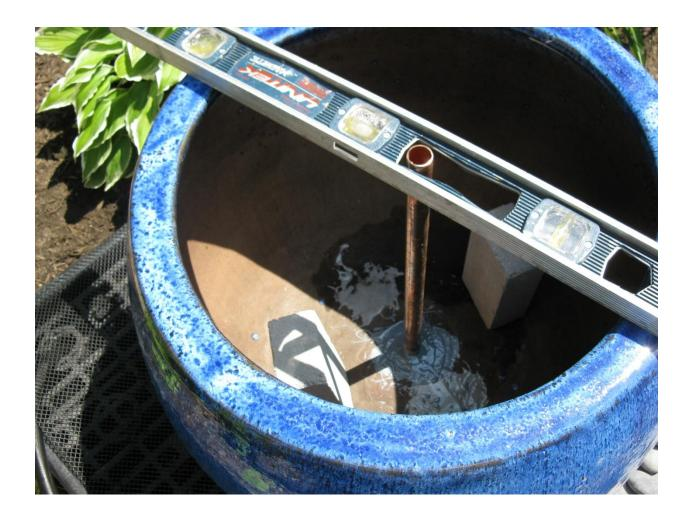
Once the epoxy dried I checked again for level, shimmed level if needed, and then filled the basin filled with water. Test again.
