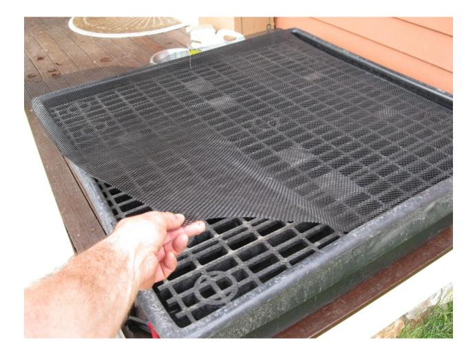
The basin will house the reservoir water pump, some pipe and other connections and will be full with water.
