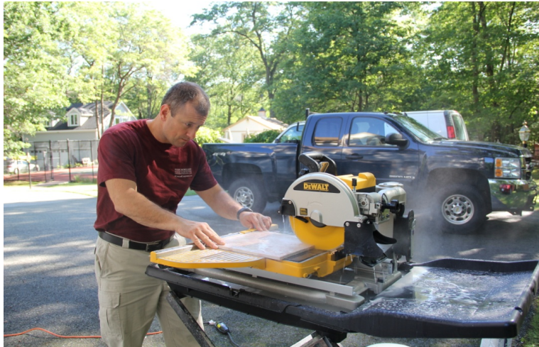
Photo: Installing tile For AConcordCarpenter TV Show [DEWALT product placement]
